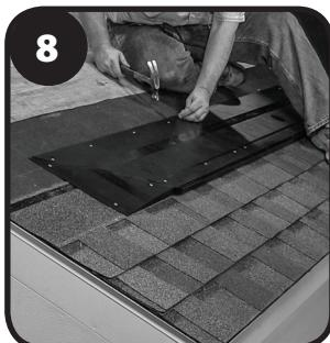
Align lower front edge of vent with exposure edge of shingle.
