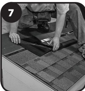
Install DA-4 over the slot using the termination method previously selected in step 1.
