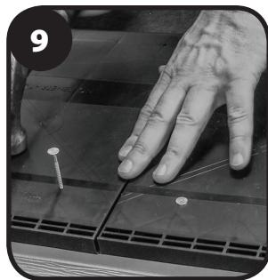
Fasten the DA-4 through the 10 reinforced nail holes using the 2½" ring shank nails provided. Leave ¼" gap between each vent to allow for expansion in hot weather.
