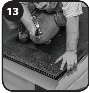
Align starter and first course shingles with shingle stops on the DA-4 to ensure top vent openings are not covered.
