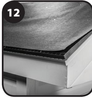
Install underlayment on top of the DA-4. This must be placed under the next layer to ensure roof drainage goes over the top of the DA-4 vent.
