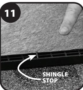
Align bottom edge of underlayment with shingle stops on the DA-4 to ensure top vent openings are not covered.
