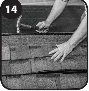
Install starter and first course shingles over installed underlayment. **Do Not** nail into the ventilation slot area.
