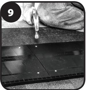
Fasten the DA-4 through the 10 reinforced nail holes using the 2 1/2" ring shank nails provided. Leave 1/8" gap between each vent to allow for expansion in hot weather.
