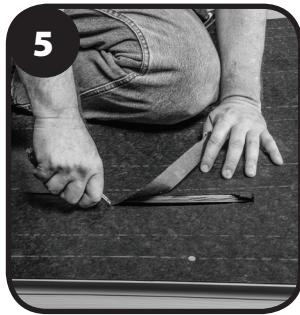
Install underlayment on the roof deck a minimum of 18" up deck from drip edge covering the area where the DA-4 will be installed. Remove underlayment that covers slot.
