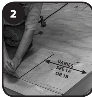
**Metal drip edge must be installed before installing the DA-4.** Using a tape measure and chalk line, mark the decking for a 1" wide ventilation slot.
