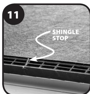
Align bottom edge of underlayment with shingle stops on the DA-4 to ensure top vent openings are not covered.
