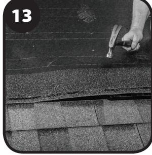
Align starter and first course shingles with shingle stops on the DA-4 to ensure top vent openings are not covered.
