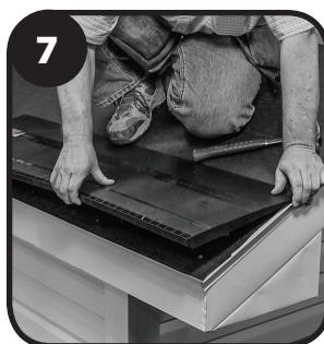
Install DA-4 over the slot using the termination method previously selected.
