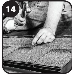
Install starter and first course shingles over installed underlayment. **Do Not** nail into the ventilation slot area.
