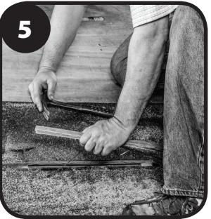
Remove cut decking along with any shingle or underlayment to clear slot. **Do Not** cut through rafters. **Do Not** over cut the slot in length or width.
