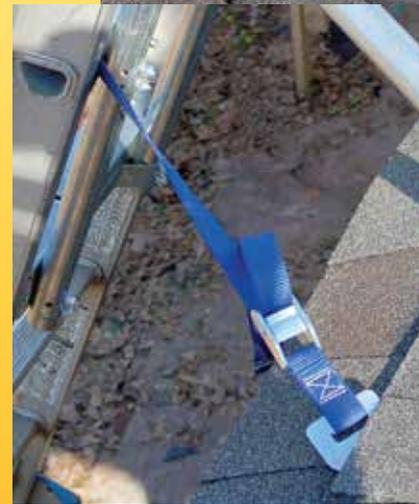
Improve job site safety by securing extension ladders and TranzSporter tracks sections using the Roof Zone Ladder Anchor. Prevents extension ladders and track sections from lateral or side to side movement.
