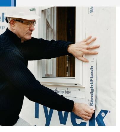
How it works: DuPont™ StraightFlash™ is designed to protect the heads & jambs of rectangular windows and doors from water intrusion.
